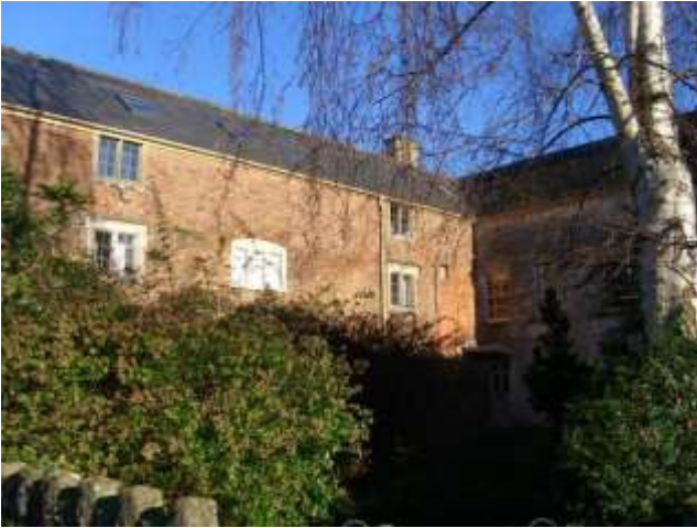
Garden of Apsley House, High Street
