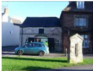
Coach House to North of former Crown and Anchor, now a pharmacy
