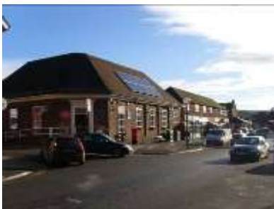
Town Hall and Post Office looking South
