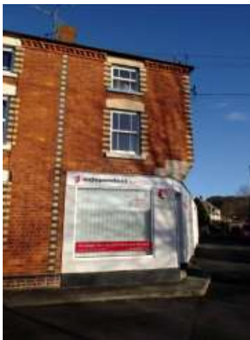
Brick and stone details, 31, Gloucester Road
