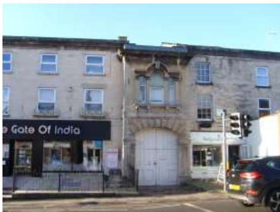
18th and 19th century limestone buildings, High Street
